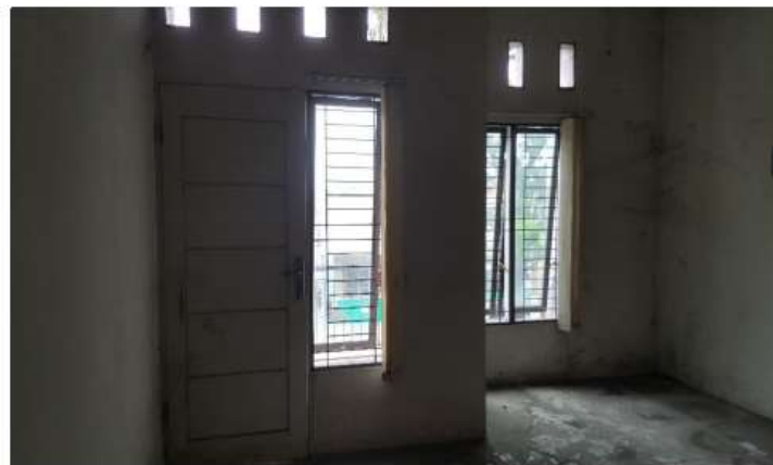
Gambar 3. Tampak Area Kafe Lantai 2
